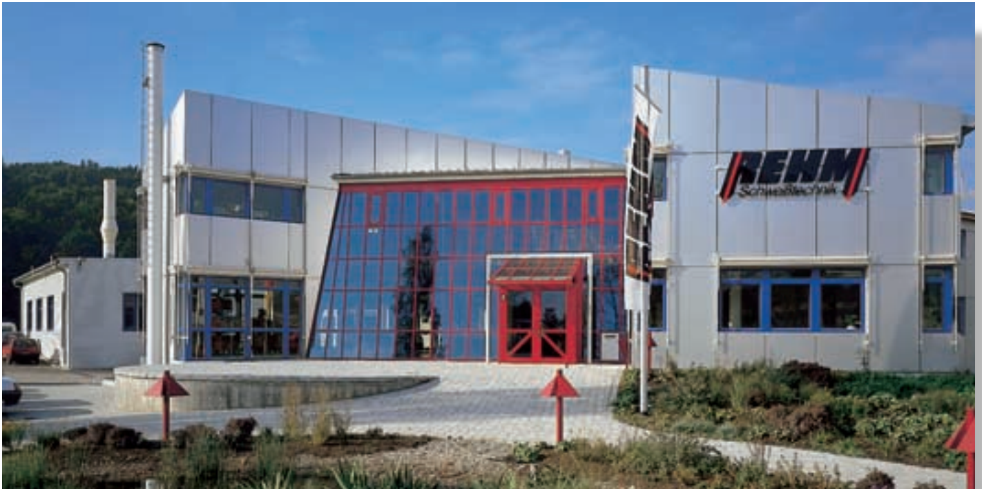
REHM welding technology in Uhingen
